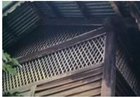
Fig.1: Woodcarving as ‘ Jejala ’ above the wall, below the roof, for ventilation purpose.
