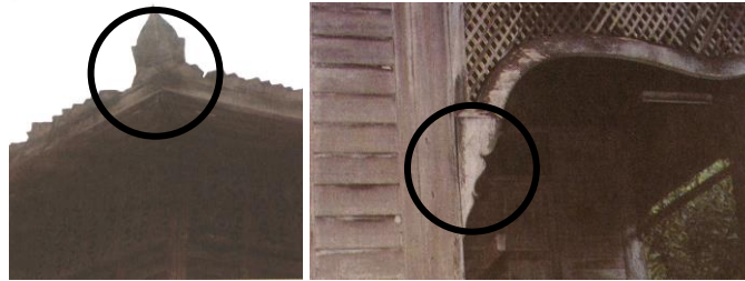
Fig. 4: Above left: End of the roof's pemeles (barge board) shaped like the tail of a duck. Above right: Siku Keluang (bat's elbow) a nickname for the wave shaped motif at the pillar, which functions to strengthen the joint between the pillar and the horizontal beam that support the roof.
